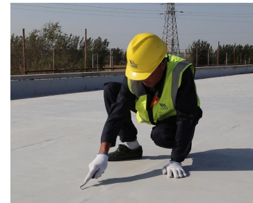
9. Seal Waterproofing sheet
