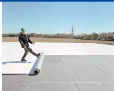
4. Pre-apply TPO Waterproofing
