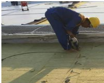
3. Pave Insulation Panel
